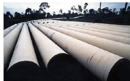
Yadana pipeline during construction
